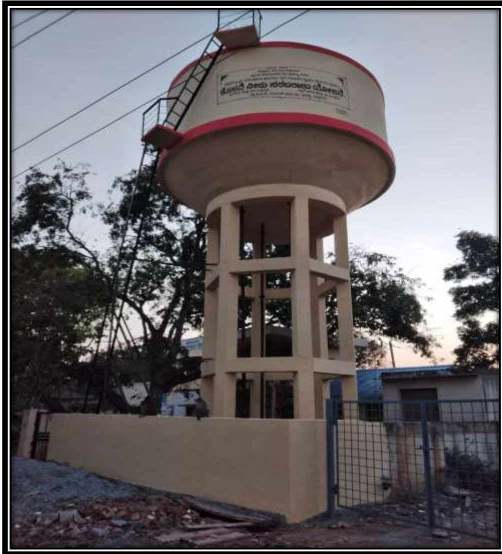
Over Head Tank constructed in Haragadde Cluster Bangalore Dist.
